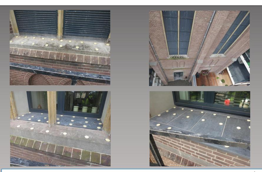
On the east side of the chapel, six window ledges were cleaned and treated with 小島 *Bird Free* as shown above.
