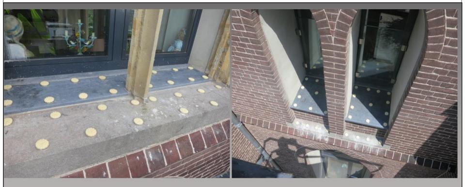
A total of eight window ledges on the west side of the chapel were treated with 小島 *Bird Free.* The recessed ledges, which offer more shelter for pigeons, were treated as shown above.
