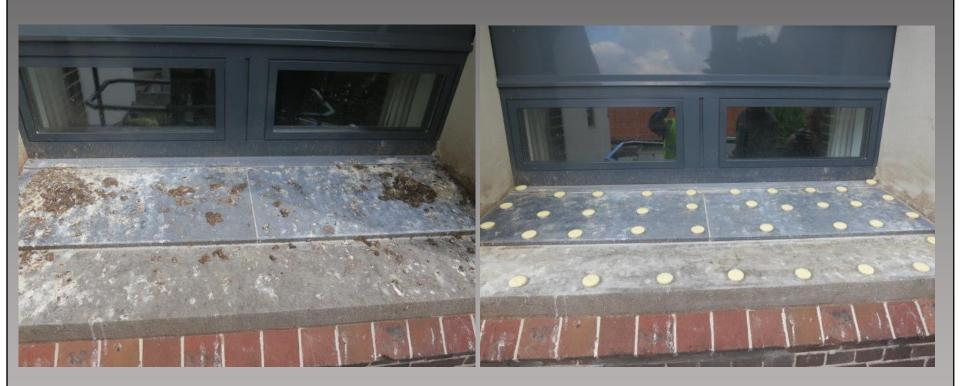
On the west side of the chapel, the window ledge to the south was severely infested (above left). This was treated with 小島 *Bird Free* as shown above right.
